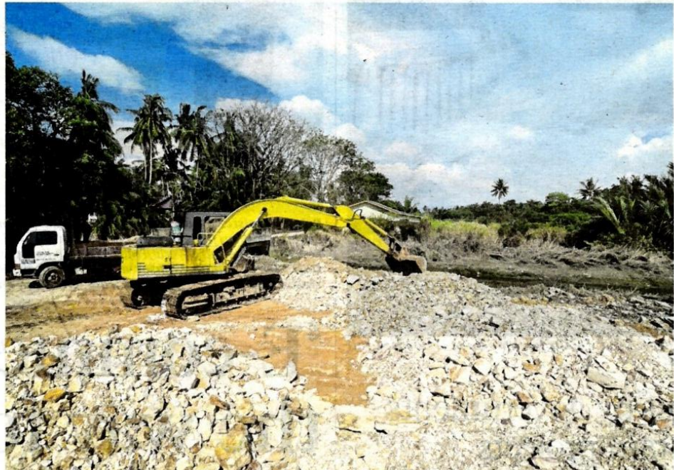
An earth-digger piling rocks to build a bund to face tidal king tides expected to hit Kampung Batu 5, Kapar, Klang, yesterday. Pic by Muhammad Sulaiman
